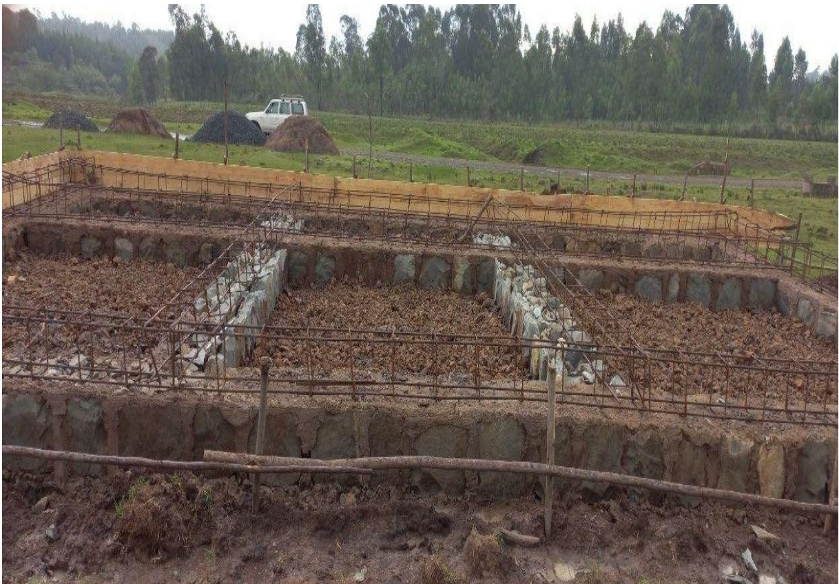
The water management office
