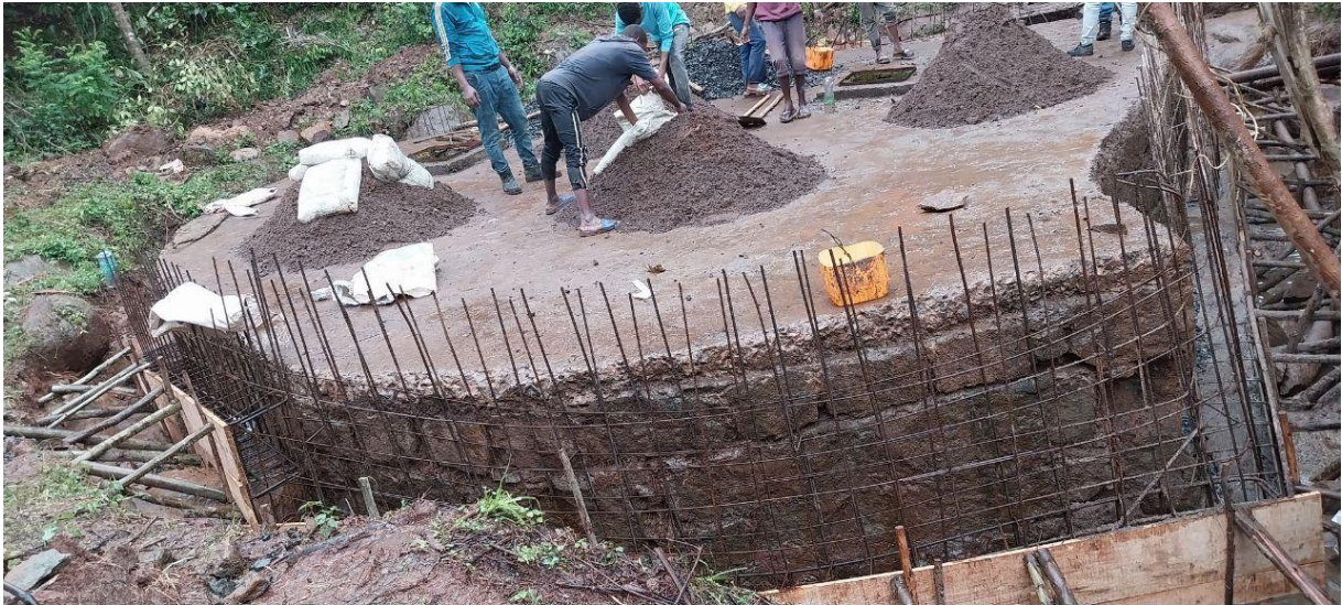
The wet well construction: the captured water flow to wet well and treated there before pumping to the reservoir.
